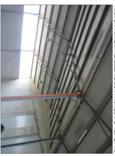
N. 24 CARRATE IN REALIZZATE CON PROFILO IPE "120" E PROFIL A "L"
