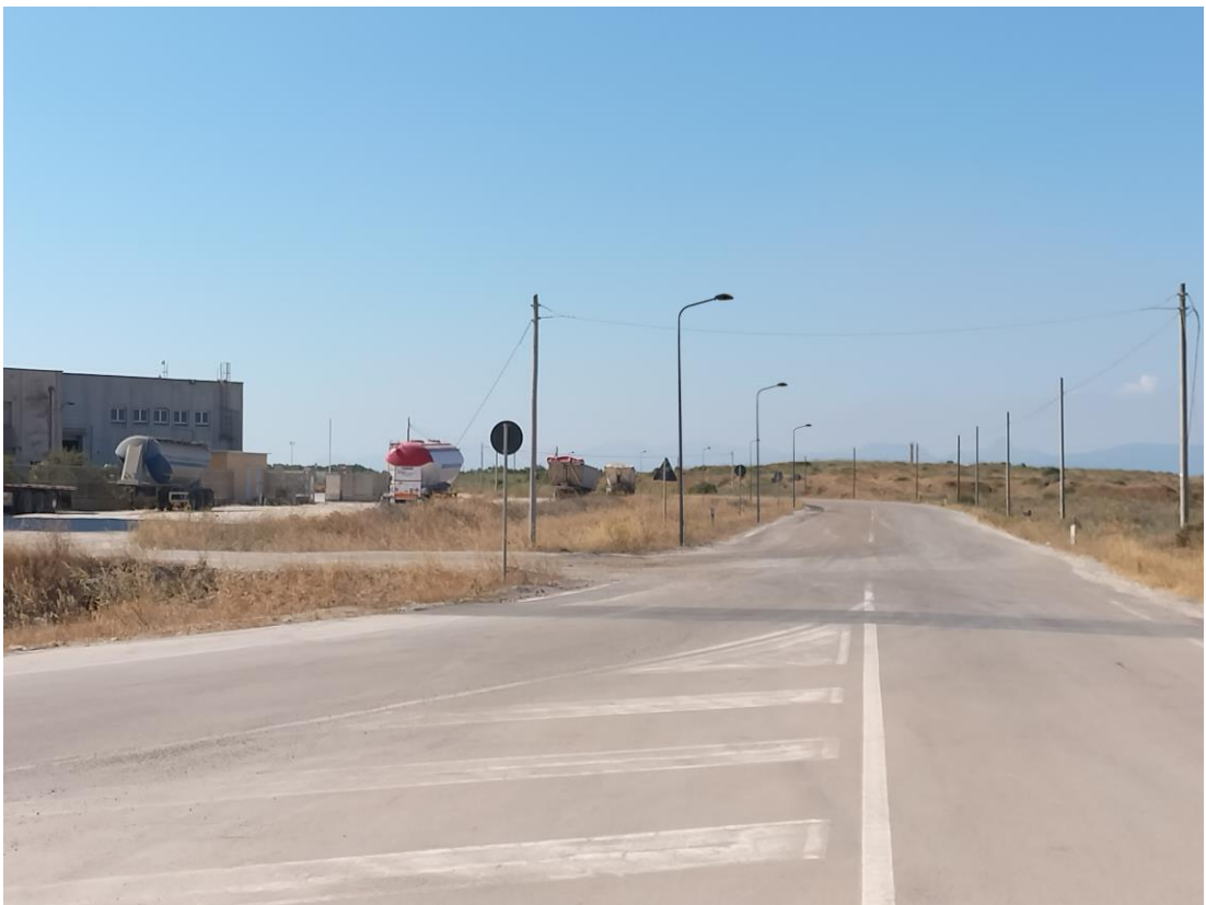
Vista 1 – Via Abbarossa – Post intervento
