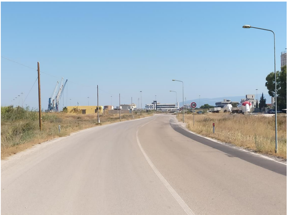
Vista 2 – Via Abbarossa – Post intervento
